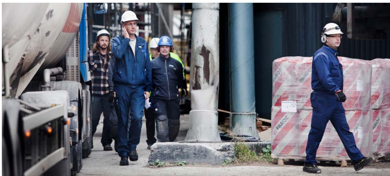
Inspections in conjunction with preparations prior to upgrading the evaporation plant at Vallvik. From right: Michael Bülow and Tord Andersson (Vallvik), Johan Sjögren (Instrument Montage), Roger Persson (Perex) and Heimo Turula (Ukitig).
