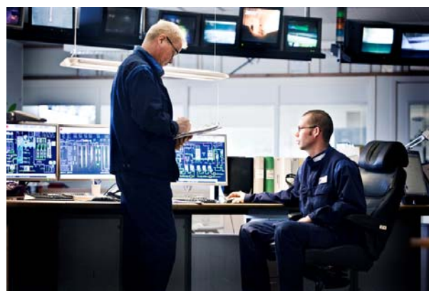
Most of the mill is controlled from the operations centre at Vallvik. Berndt Åkerdahl on the left is an operations engineer and Robert Jansson is an operator at the recovery boiler.
